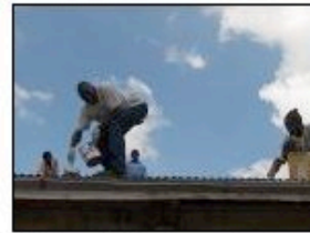
Mutuku painting the roof of the dispensary
